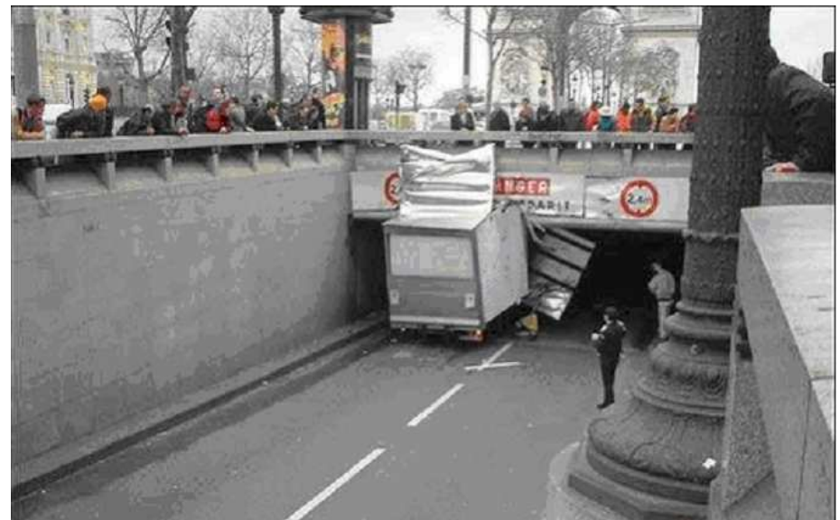
The top of a truck is given a shaving because of a mismatch between the height of the truck and the clearance of the overpass.
