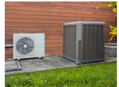
The outside equipment for a typical residential heat pump.
