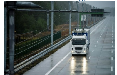
Conductive overhead catenary system
