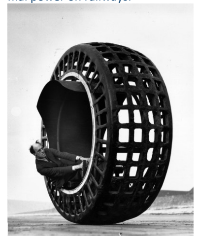
17. The DYNASPHERE - an electrically-driven wheel, capable of speeds of 30mph, invented by Mr. J. A. Purves of Taunton and his son.
