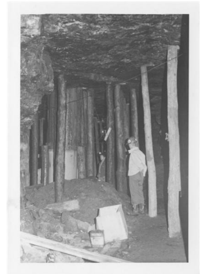
When the pillars as well as coal in the roof were removed by coal robbers after the mines were abandoned, timber pillars were placed in for support. These supports were never intended to be permanent. Their purpose was to keep the roof from falling on the robbers while they worked.
