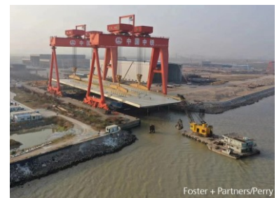
Cranes lift the 3,500-tonne completed Slussen bridge onto pontoons at a shipyard in Zhongshan outside Hong Kong.
