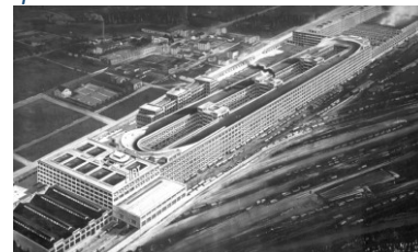
The Fiat View of Fiat Lingotto Factory in Torino, with a test track on the roof, completed in 1923.
