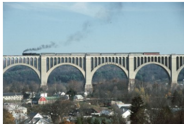
The Nicholson Bridge, officially the Tunkhannock Creek Viaduct, is still in use for the Norfolk Southern Railway. It was designed and built by DL&W staff and completed in 1915. It is among the world's largest concrete bridges ever built.
